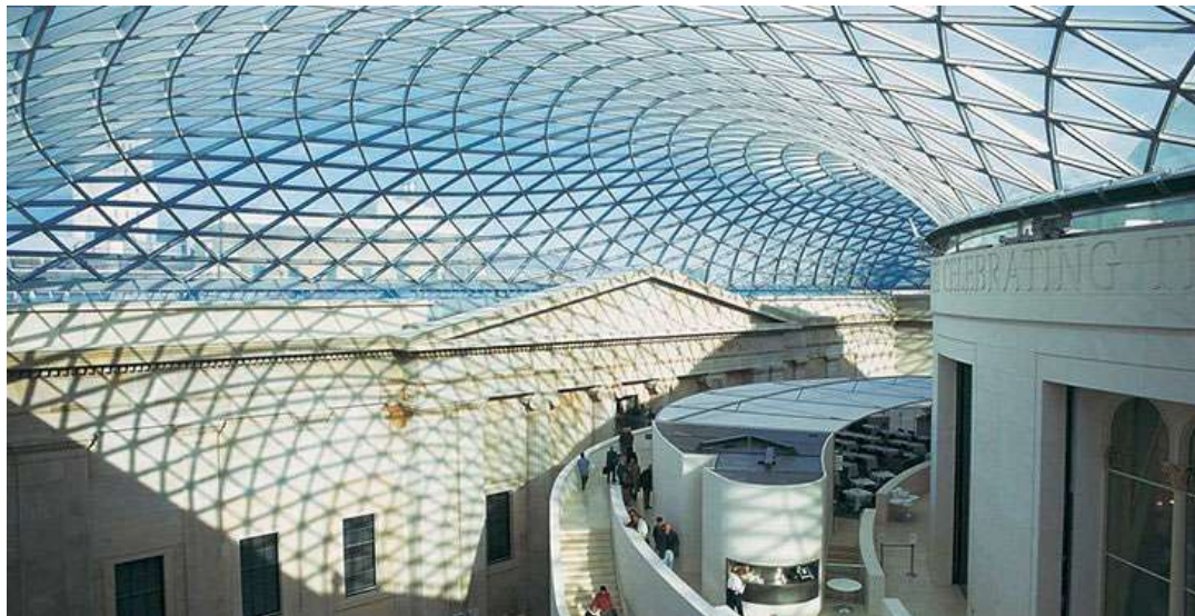
the British Museum courtyard, covered with grid shell
