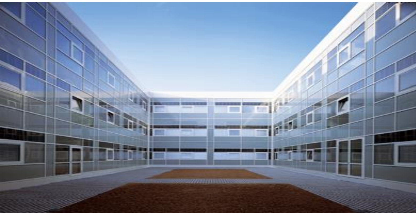
Hospital for accidents, Murnau Gartner AG
