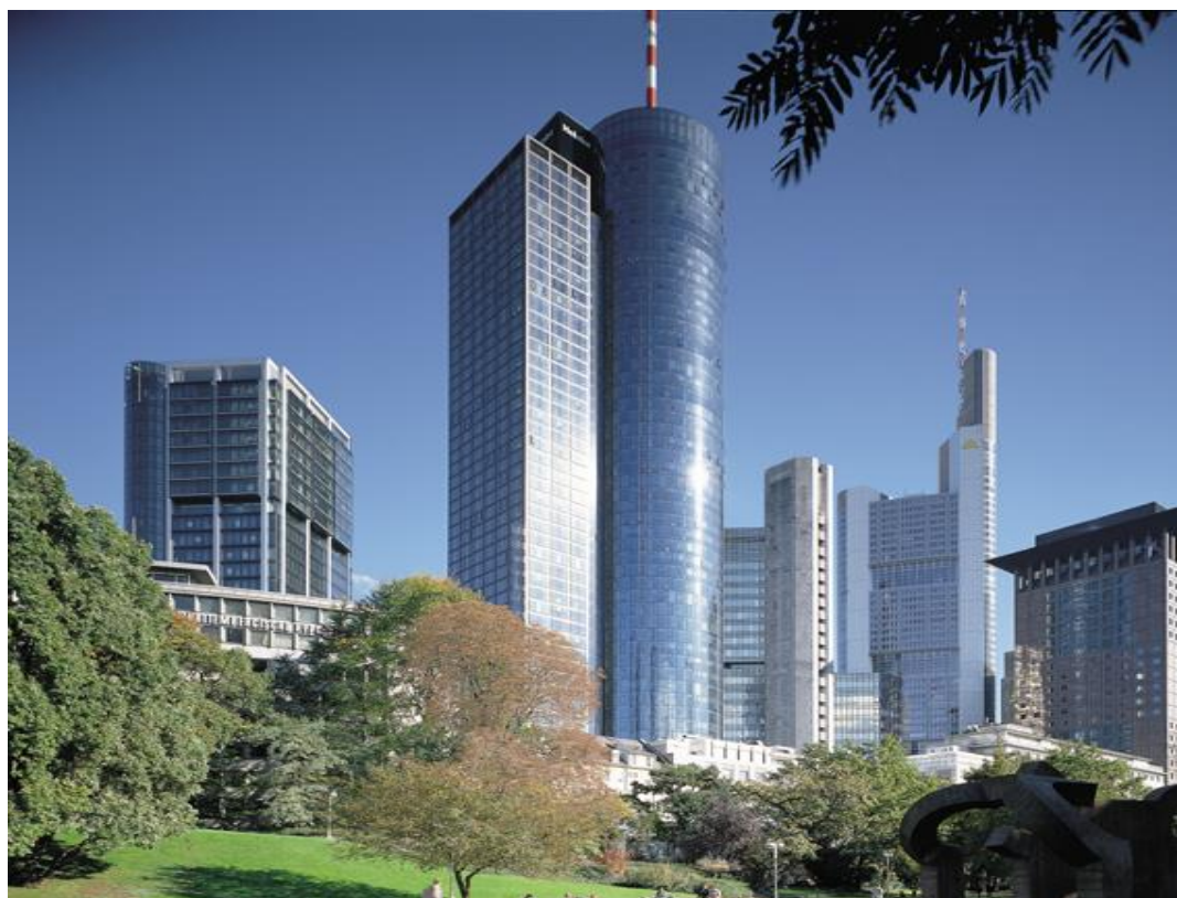
Maintower, Frankfurt Gartner AG
