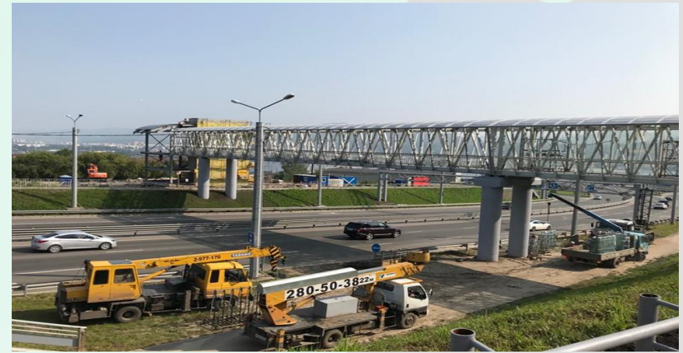
Installation of superstructure on-site
