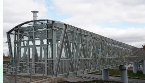
Krasnoyarsk Construction period 2019 - 2020
