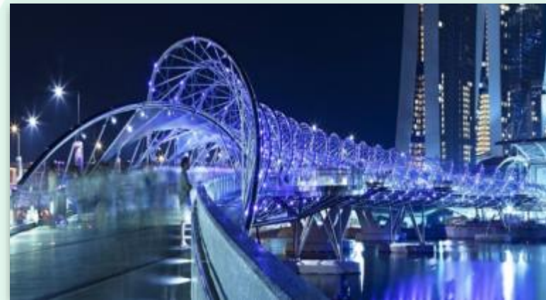
Helix Bridge, Singapore
