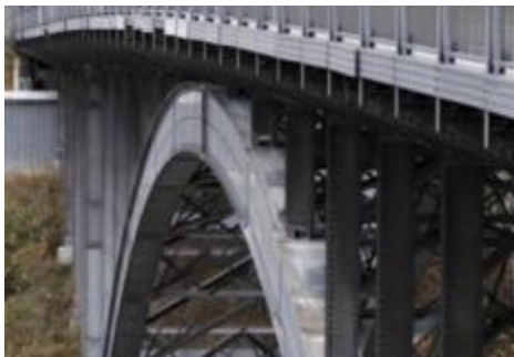
The world's first 100% aluminium bridge was built in 1949 over Saguenay river in Canada
