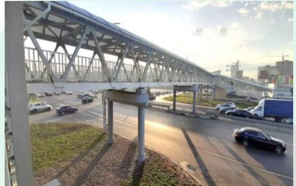
Красноярск In operation since 2018
