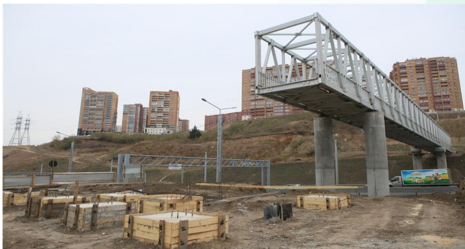
Installation of superstructure on-site
