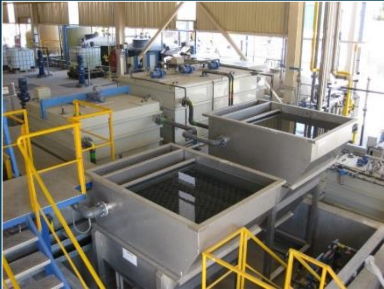
ZLD plant Sulphates and Fluorides treatment
