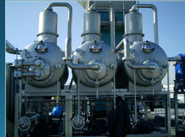
ZLD plant Triple stage evaporator
