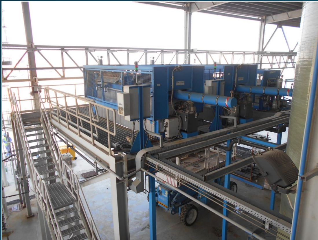
PURAL ZEROZERO Lamella settlers battery
