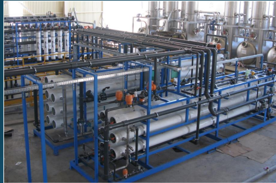
ZLD plant – U.F. and R.O. view
