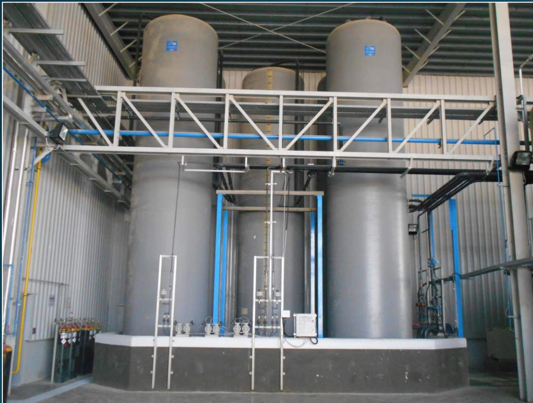
PURAL ZEROZERO Waste water buffer Tanks
