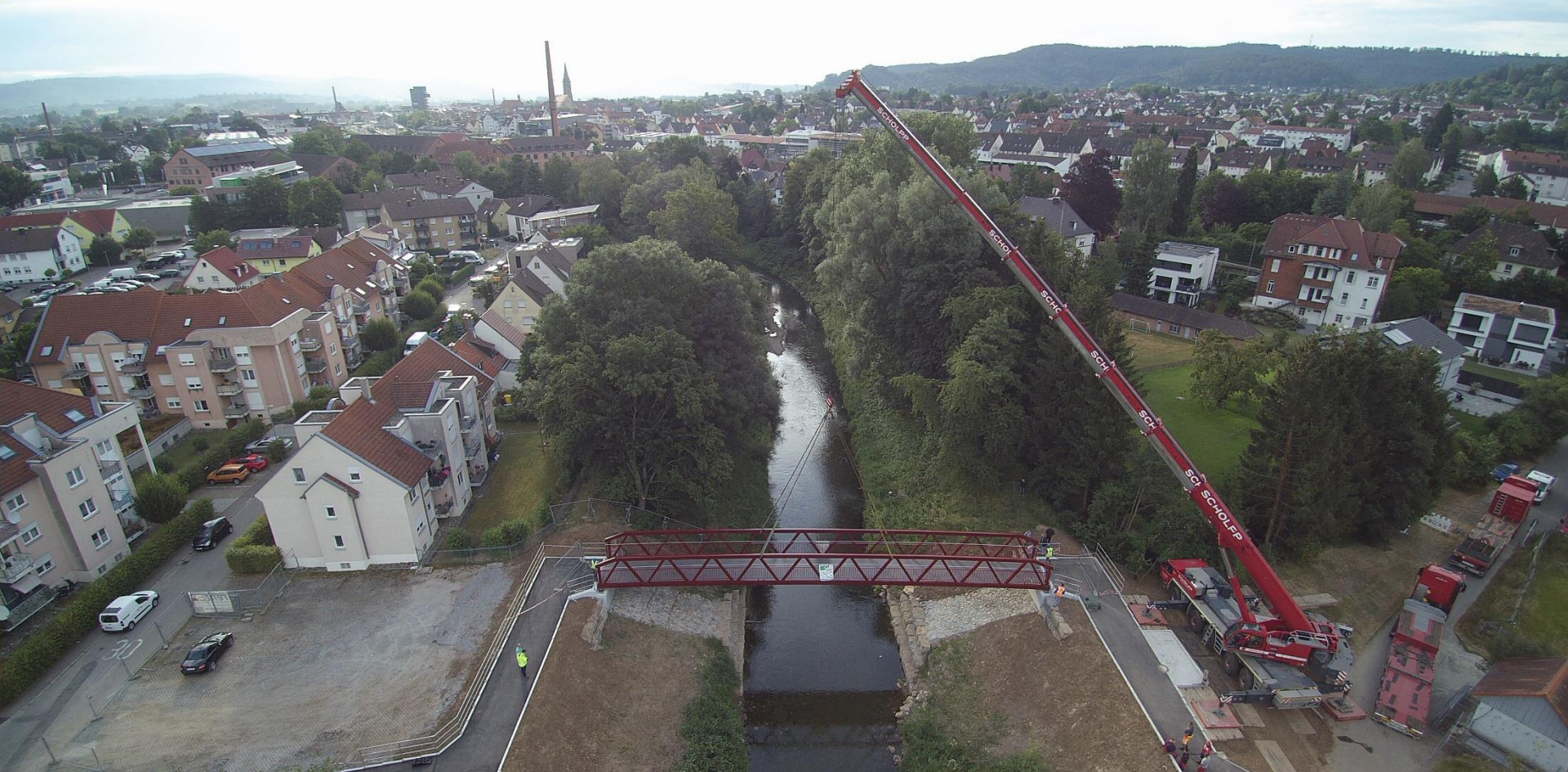
Pedestrian and bicycle bridge in Schorndorf span width: 32 m, width: 3 m
