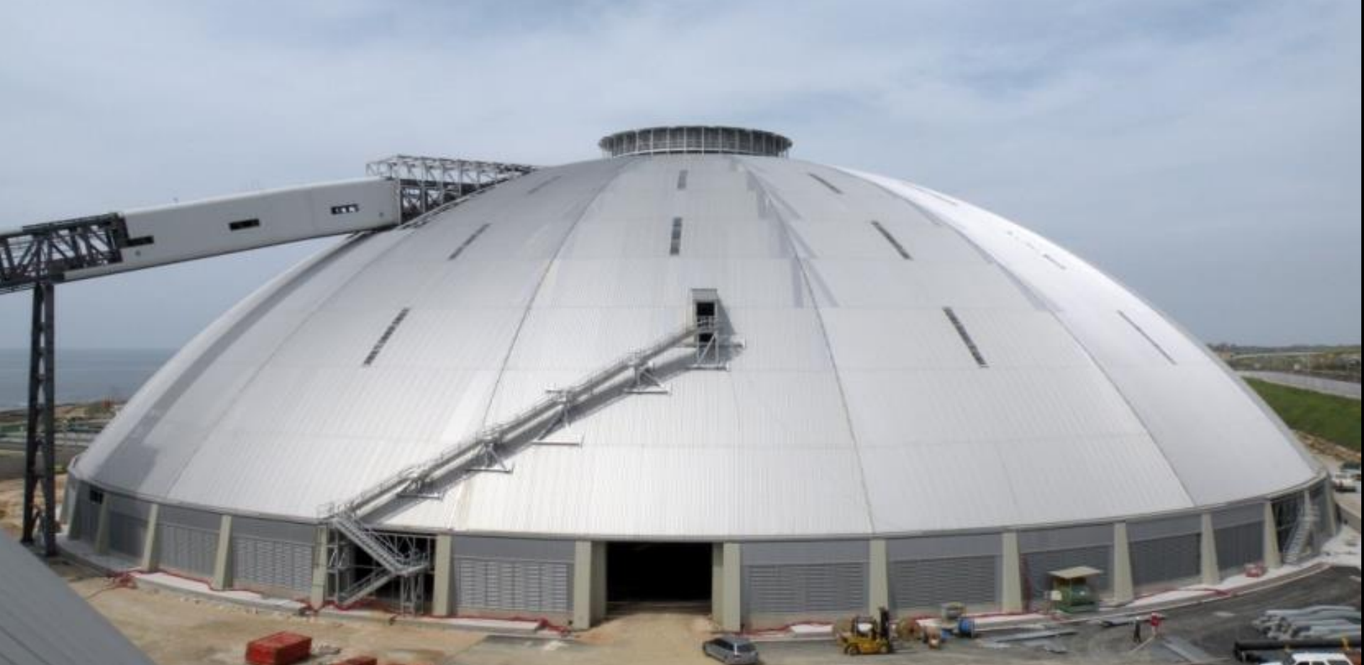
Two Twin Aluminum Domes of the Enel Plant in Civitavecchia (Italy), Aluminium Roofing and substructure (diameter 144 m and 49 m height)
