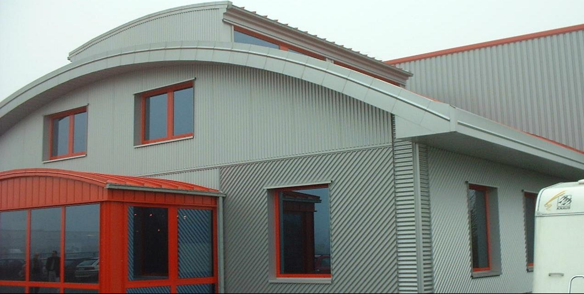
Facade made of roll-formed profiled panels Corrugated profiled sheet, coil-coated
